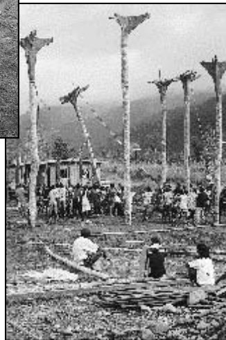
Right - Kokoda villagers erecting the platform used in the opening ceremony. Each village in the district cut and decorated a tree, carried it to the site and then, in one afternoon, with much ceremony and straining set them up as shown. Jungle vines were used to pull the trees upright and smaller vines then used to lash the platform in place.
