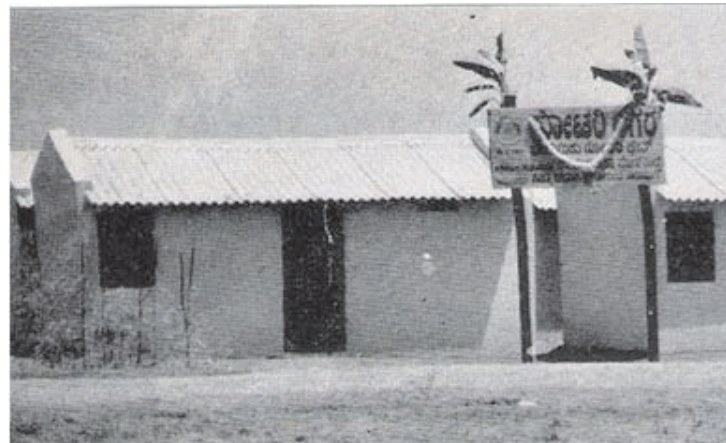
Houses constructed and donated at Rotary Nagar in Kodichikkanahalli.
